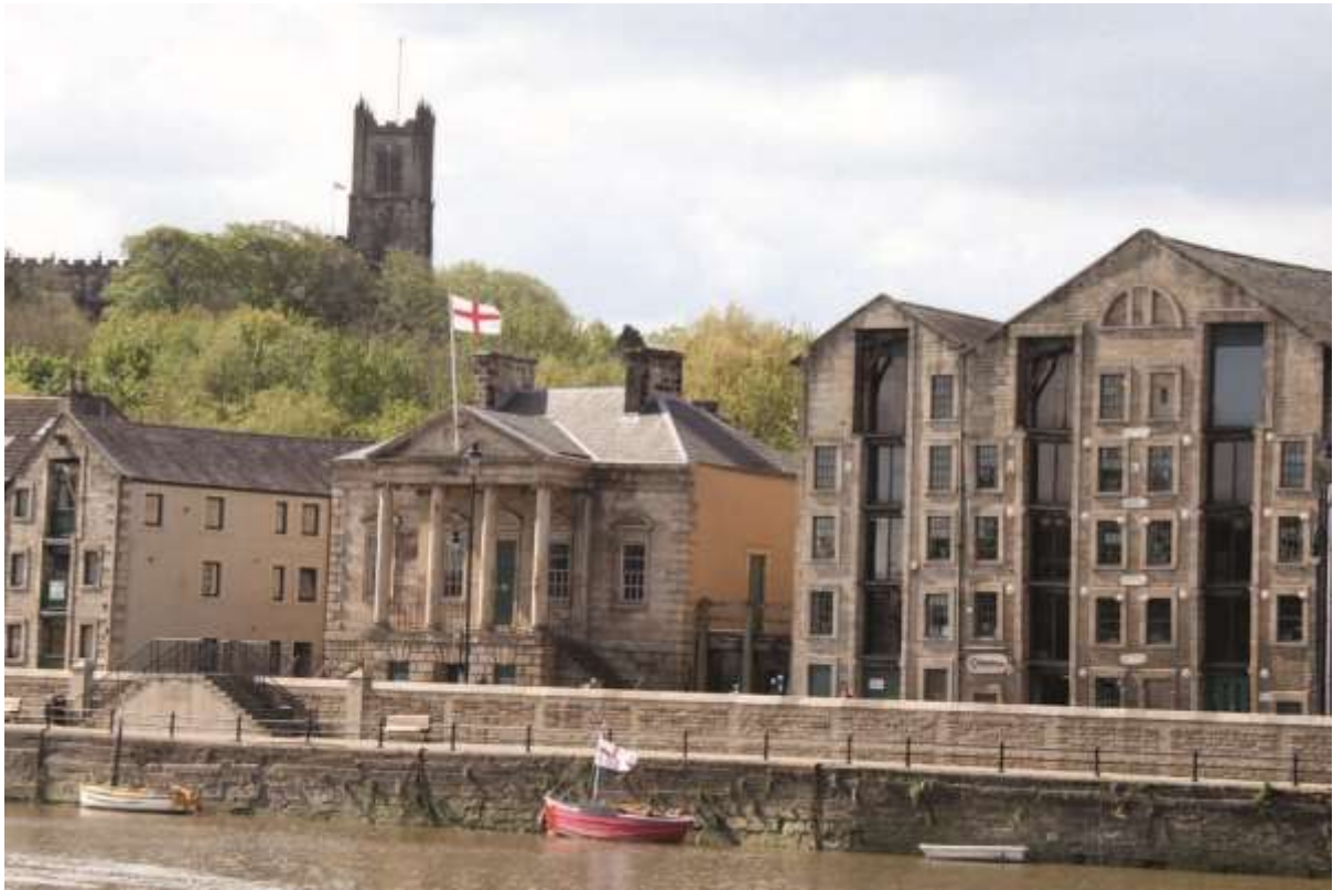
Customs House, Lancaster designed 1764 by Richard Gillows, Foster's house and warehouse is to the right.
